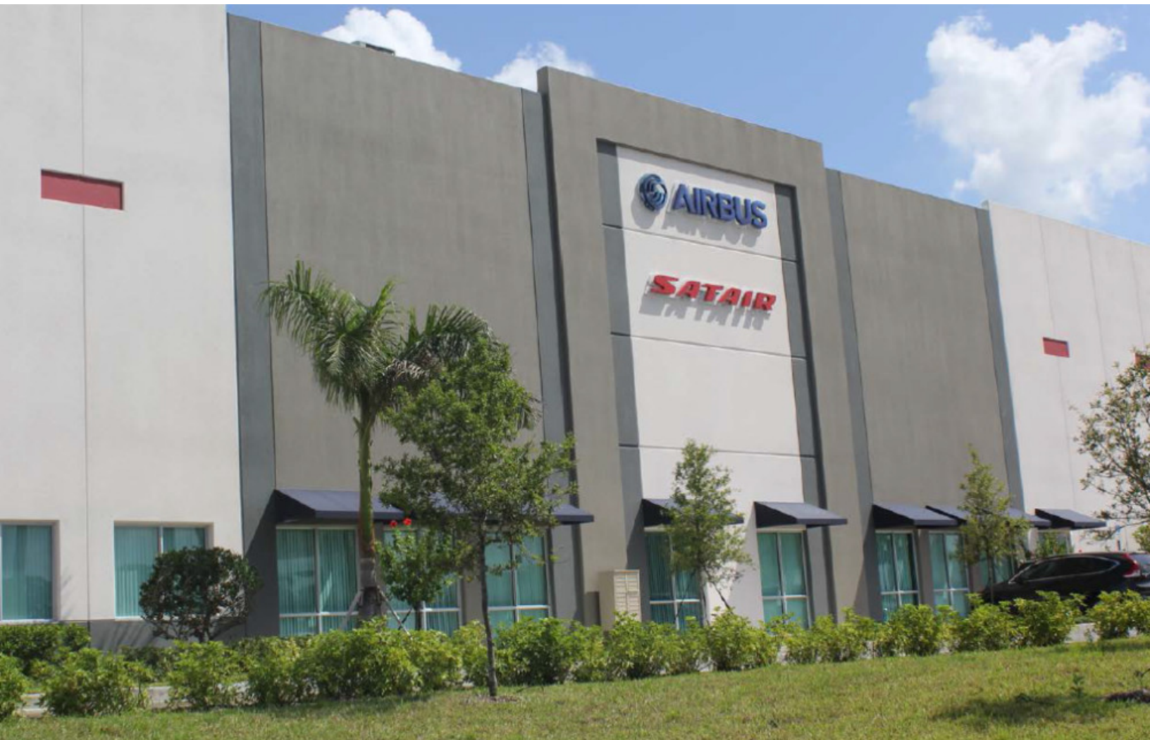
New Satair Group Miami facility
